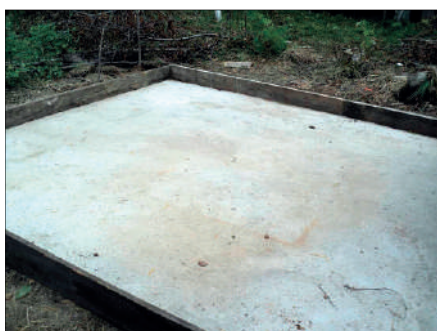
Preparation and the pouring of the concrete pad.
